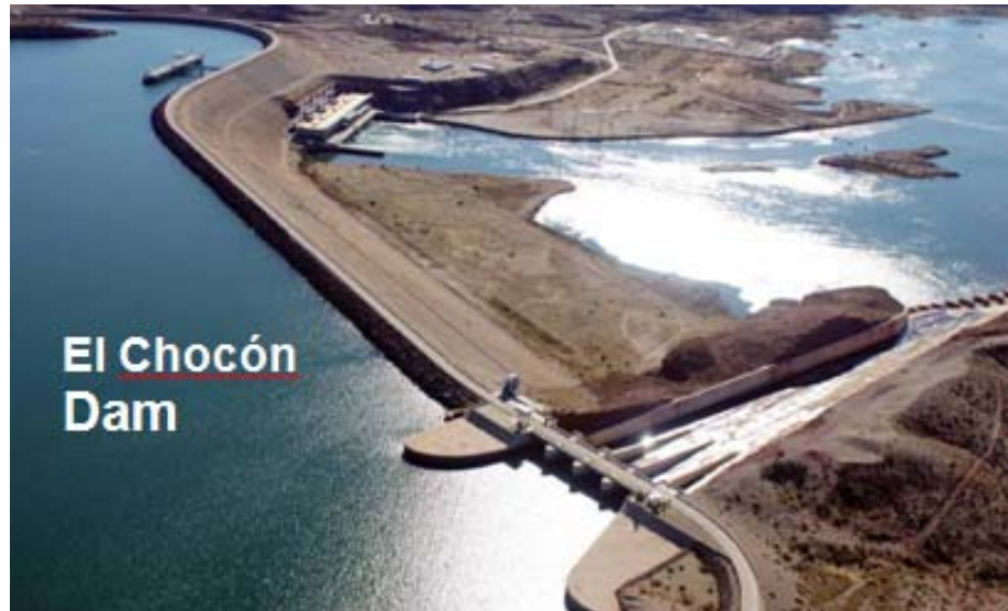
Figure 6. Aerial view from right bank
